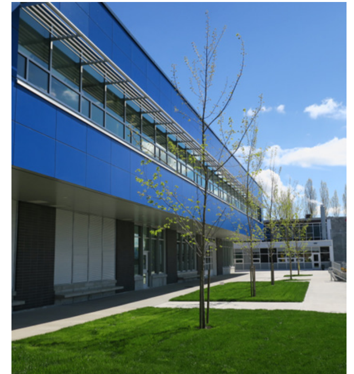
Alpha Secondary School New Wing (Seismic Partial Replacement)
